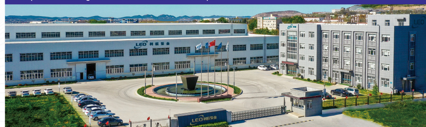
Pump Manufacturing Base for Petrochemical Industry
